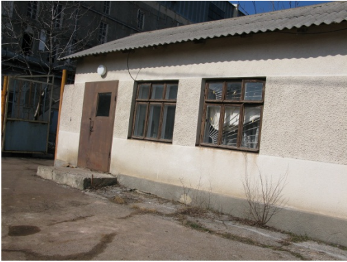
This large production building was used for spirit production (old technological equipment is still inside):
